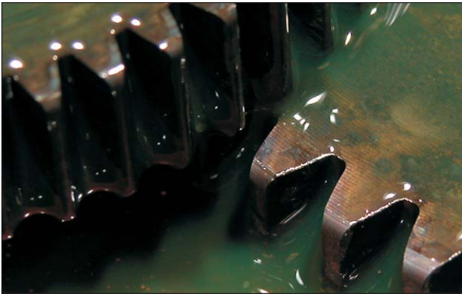
Proper oil level - just below top of output gear
